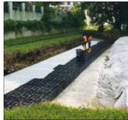
Housing development, Singapur (SG)
