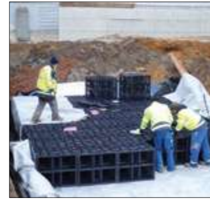
Industrial building, Tumeltsham (AT)
