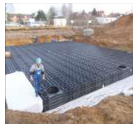
Industrial building, Merseburg (DE)
